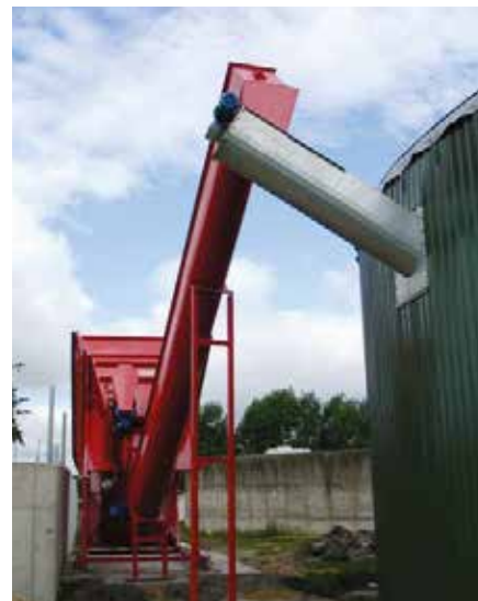
AISI 316 L, Stuffing auger for feeding into a biogas reactor, the auger works as a water lock, thus keeping the gas inside the reaktor.
